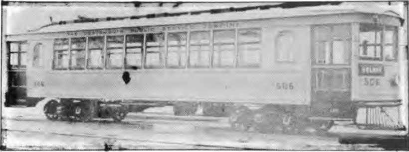
Curved-side streetcar No. 506, as seen from right (above) and left-hand sides. These cars were orange or yellow-orange with grey roofs. On interurban service, the 500s did not ride as smoothly as their Kuhlman-made predecessors.
