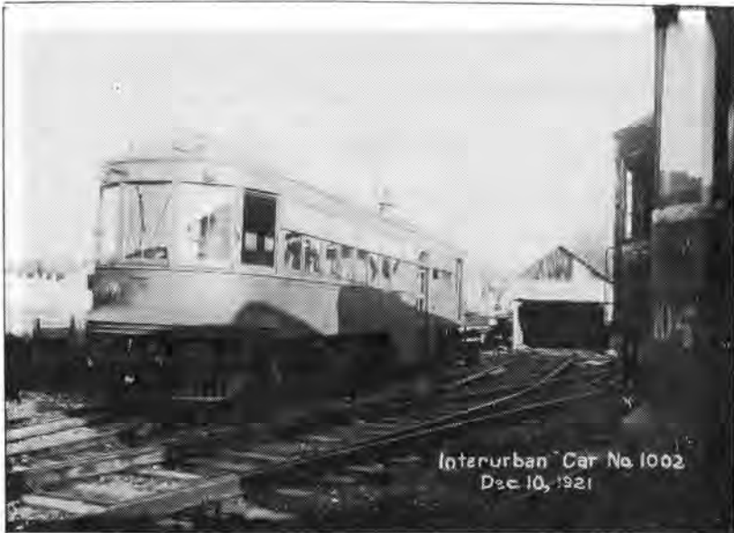
Ohio Valley Traction Co. car No. 1002 at car barn yard behind Second Street, December 1921. CITY OF PORTSMOUTH, 1921 COMPANY AUDIT
