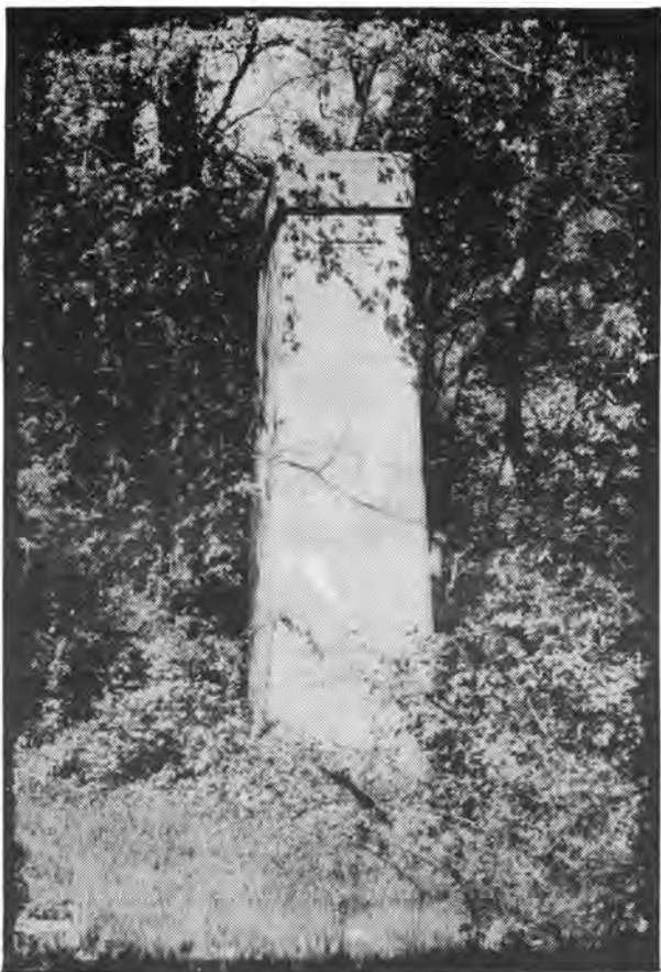
One of two piers, built by Ohio Valley Traction Co. and dated 1915, still loom today amid brush and trees on the west bank of the Little Scioto River at Sciotoville as a reminder of the old interurban line, which ceased operations in January 1930.
