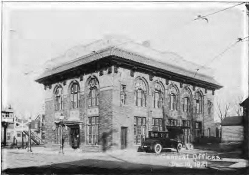
General office building and station (above), constructed in the fall of 1913, housed offices of both PSRR&LC and OVTC. Note old Norfolk & Western Railway watch tower at far left and wye service tracks. Floor plan of the building appears below. CITY OF PORTSMOUTH, 1921 COMPANY AUDIT
