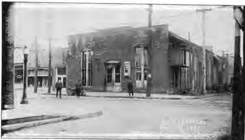
Electric substation at 10th and Offnere streets, December 1921, housed equipment supplying power to the streetcar system.
