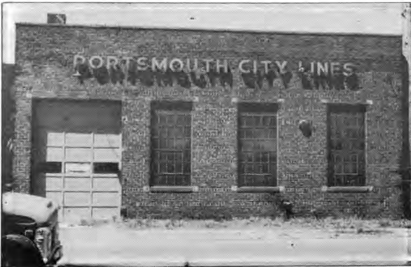
Portsmouth City Lines lettering still hangs on the east side of the former car barn shop building at Third and Madison streets in this 1986 photo. Note size of door at left. West-side wall once had four doors, and interior floor contained four inspection pits. LARRY STANLEY COLLECTION
